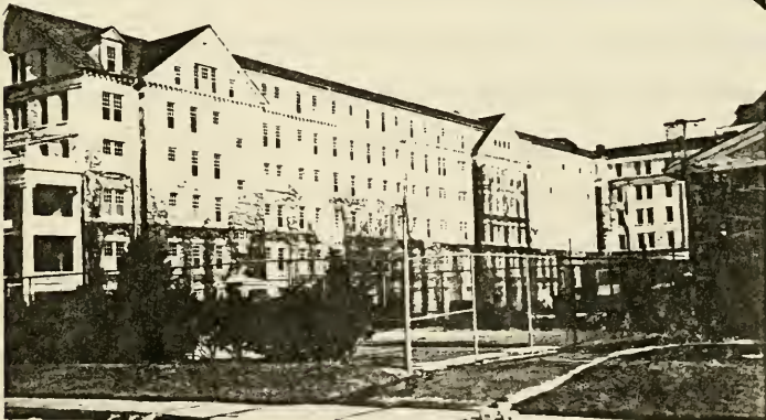
Plate 43: North Wing, South Elevation, 1985
